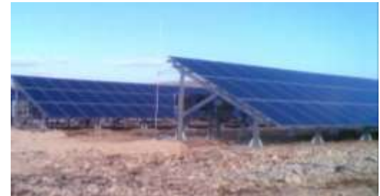
Stolac, 150 kWp Bosnia & Herzegovina
