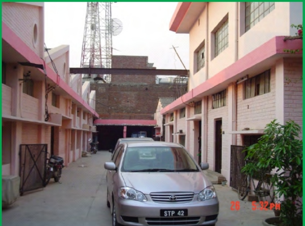
Outside Production Halls
