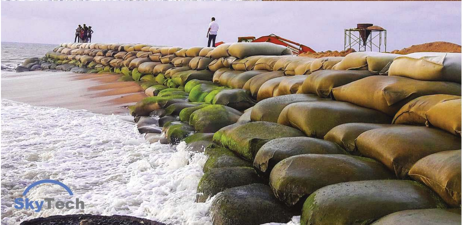
Break Water & Rivertment Project Chilaw, Sri Lanka
