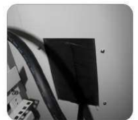
Cable entry plates with brushes
