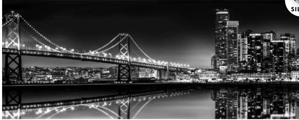
CA-12203 • ST485 • Bridge
